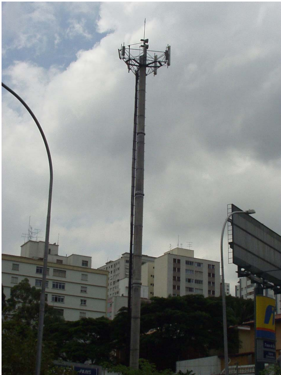
Fig. 1 – Typical pre-cast RC telecommunication tower
